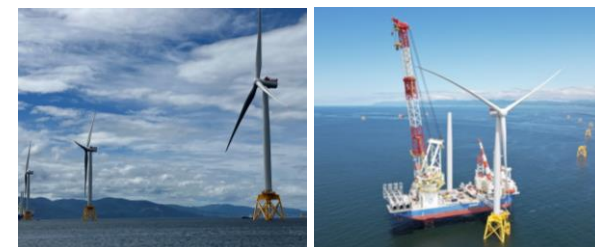
Turbine Generator Installation
